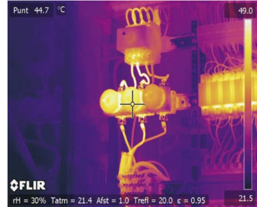
inspecting load problems at electrical cabinets of a public building (police station)
